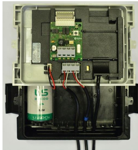
Picture 5.2 - Module installed in meter
